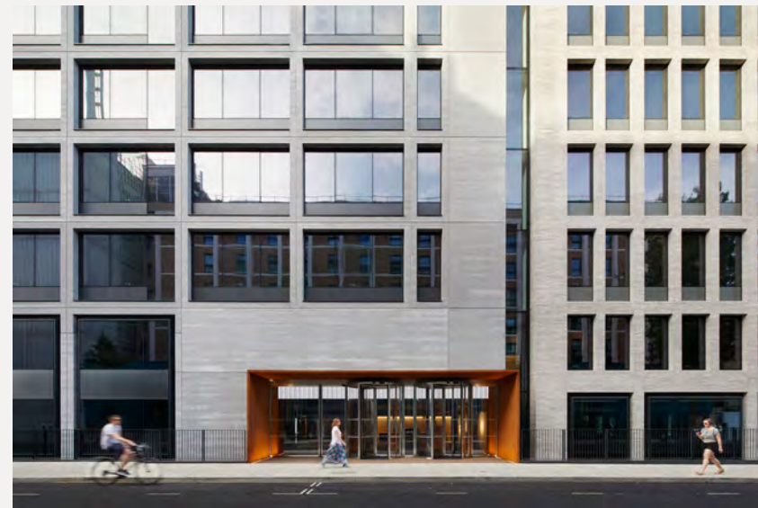
Top 80 Charlotte Street, WI entrance Above 80 Charlotte Street, WI elevation
